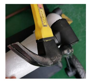
3. To assemble new caster to tube by rubber hammer, use foam to protect caster.
